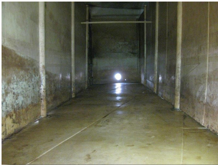
Figure 3: Skim Tank Internal Baffle Walls and Floor
